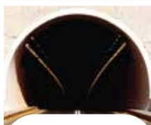
AIROLI-KATAI NAKA TUNNEL
